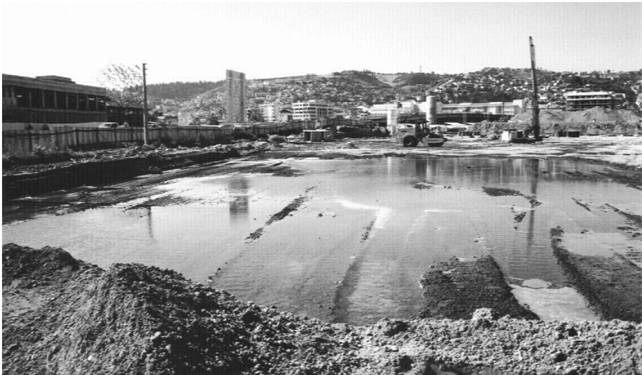
Figure 3. Ponding of water at portions of the parking structure area that were not yet treated with jet grout columns, Lot C under the preload fill is visible at the back – photograph taken the morning after the earthquake from the site border looking north
