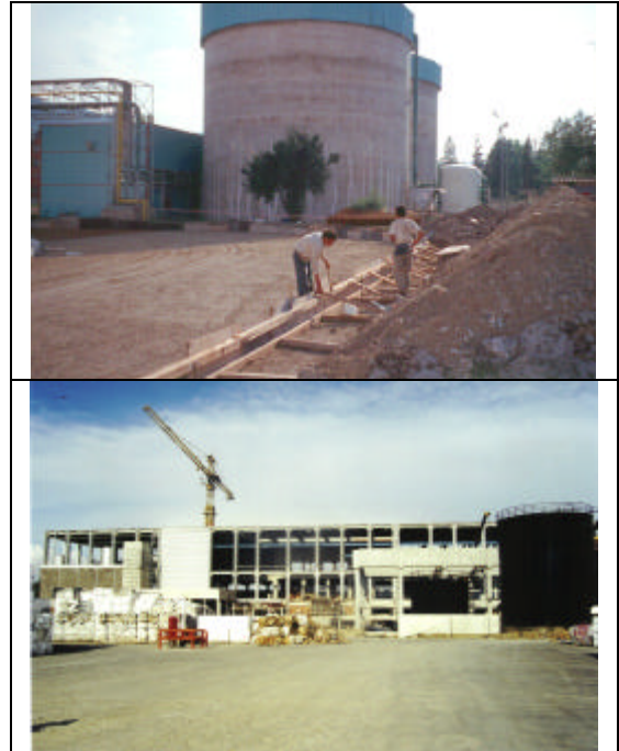
Figure 3. Water Tanks and PM3 building during construction
